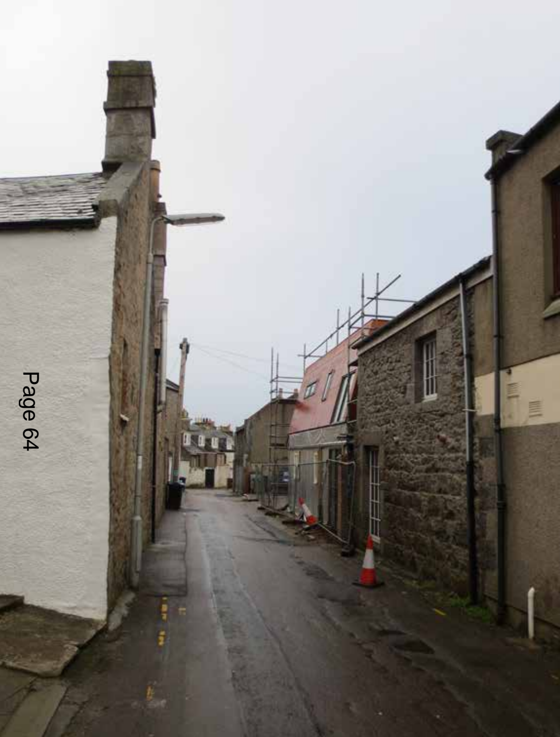
Bon Accord Lane – new mews building under construction
