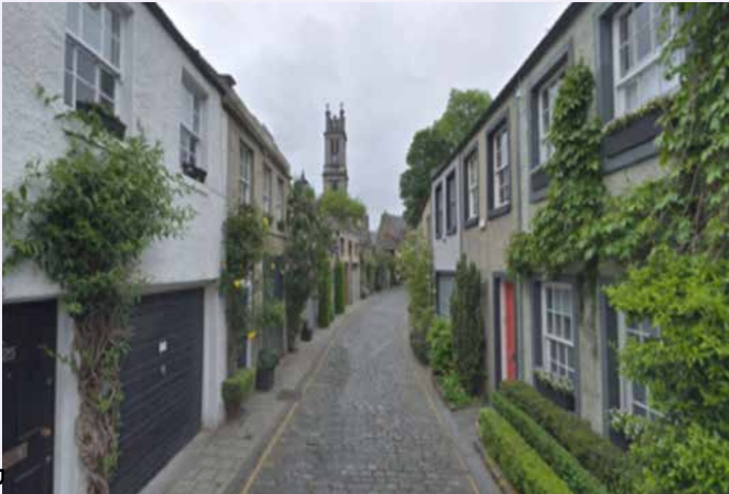
Historic mews in Stockbridge Edinburgh converted into attractive dwellings with minimal setback enabling some soft landscaping to enliven the lane
