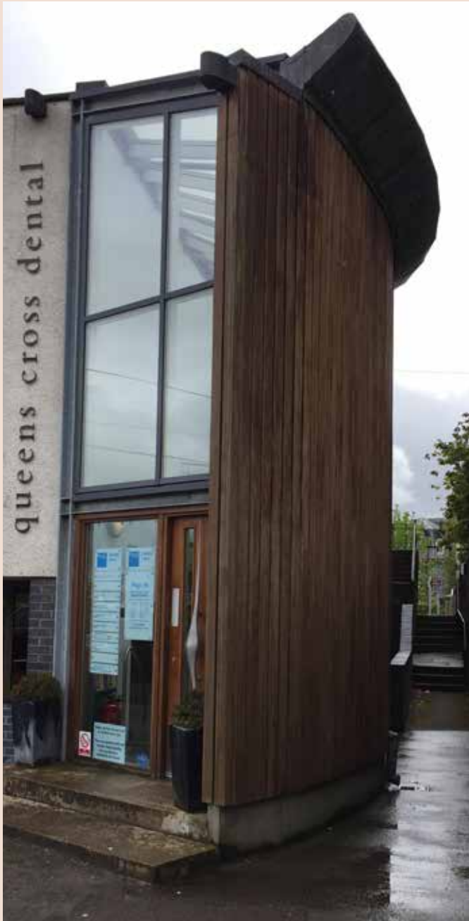
Vertical timber cladding to rear extension of Queen's Cross Dental in interesting curve design
