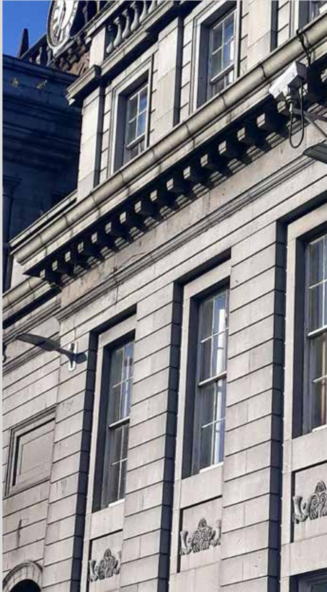
Intricate carvings, such as those on the Archibald Simpson's public house building on Castle Street (originally the North of Scotland Bank), are rare. The majority of granite façade detailing in the city is robust and elegant.
