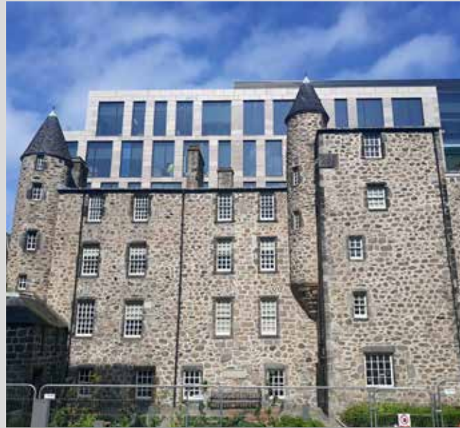
Provost Skene's House Built of granite-rubble in the 17th century it is one of Aberdeen's oldest remaining buildings
