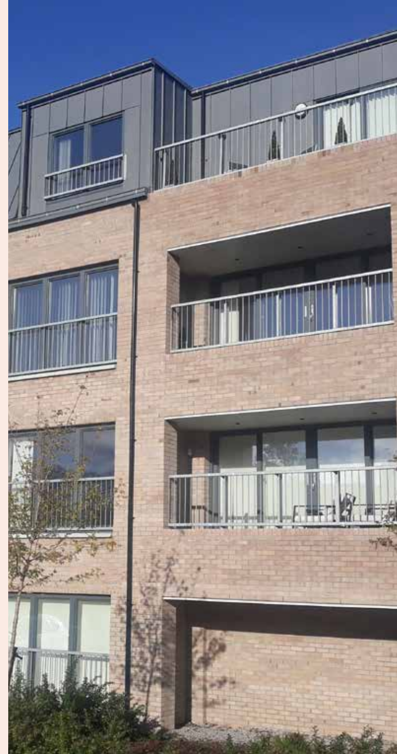
Buff toned brick used at Craiginchies offers a contemporary contrast to the surrounding granite of the tenement buildings in Torry
