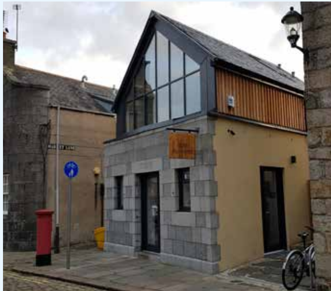
The use of glass in the upper gable of this roof extension maximises daylight receipt and minimises the extension's massing
