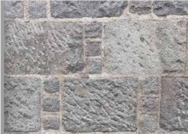
Aberdeen Bond – The distinctive coursed pattern, using a stack of three smaller granite offcuts (from the quarry sett-makers), was efficient and adds interest.
