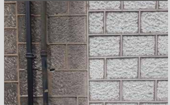
New next to old – This photo shows the importance of blockwork size in respecting context. The new granite (right) blocks are not large enough to match the existing.
