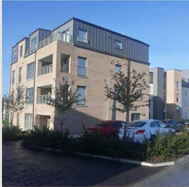
Metal cladding creates a roofscape at Craiginchies
