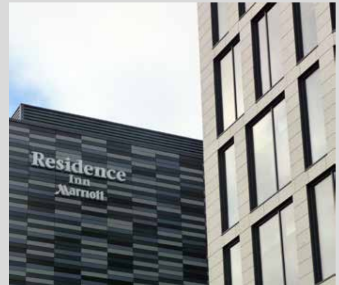
Imported granite cladding panels have been used successfully on new buildings in Aberdeen such as Marischal Square
