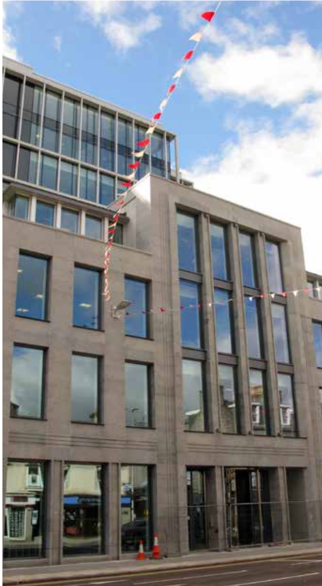
The Silver Fin The frontage faces onto Union Street, the use of light-grey granite cladding respects the street's granite heritage and colour, whilst the use of glazing in the taller element behind helps to reduce its massing
